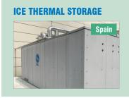
Ice thermal storage technology is used to build and store cooling when cooling demand and/or energy rates are low, which the system then uses for air conditioning or process purposes when cooling demand is high or for emergency cooling.
