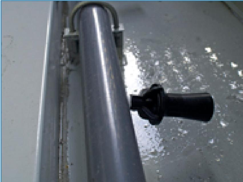
A sump sweeper piping system **increases water circulation and agitation** in the basin and is designed to be used in combination with a [filtration](#) system. It does all this:
