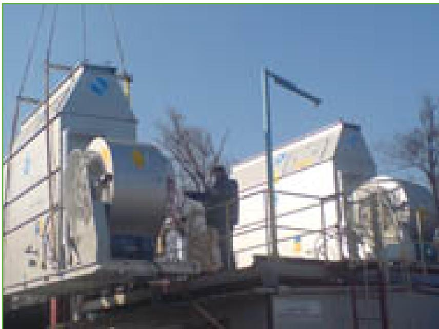
With discharge hoods, you can comply with layout restrictions by **elevating unit** discharge above adjacent walls and increasing discharge air velocity to **reduce the risk of re-circulation** in confined spaces.
